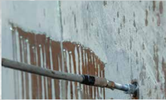
Concrete Injection
