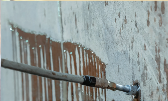
Concrete Injection
