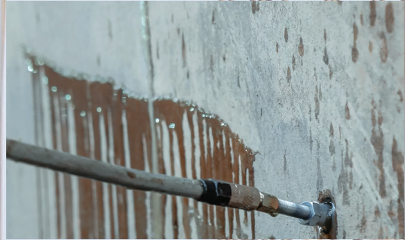
Concrete Injection
