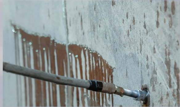
Concrete Injection
