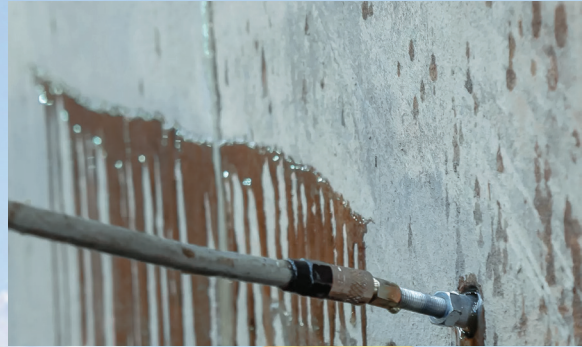
Concrete Injection
